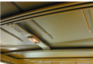
Metal roof bows center rear,
